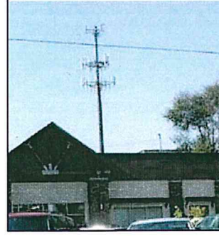
Unacceptable Monopole Macro Example
