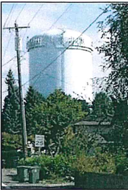
Acceptable Structure-Mounted Macro Example
