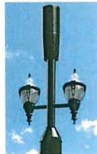
antenna to the top of the pole shall be fully concealed and integrated with the pole, to the extent technically feasible.
