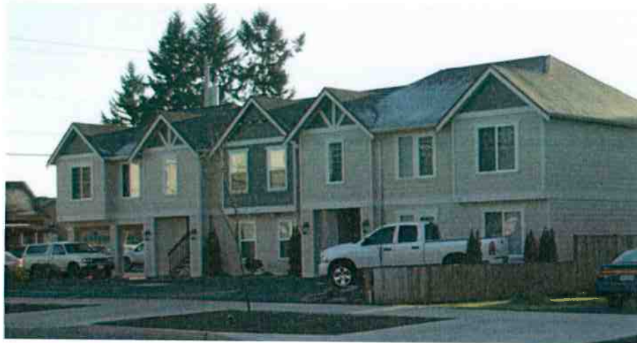
Five-plex Building; Corrin Ave SW and Bridge St SW.
