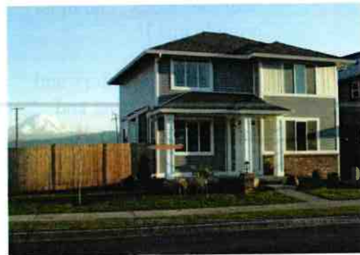
Village Green single family residence.
