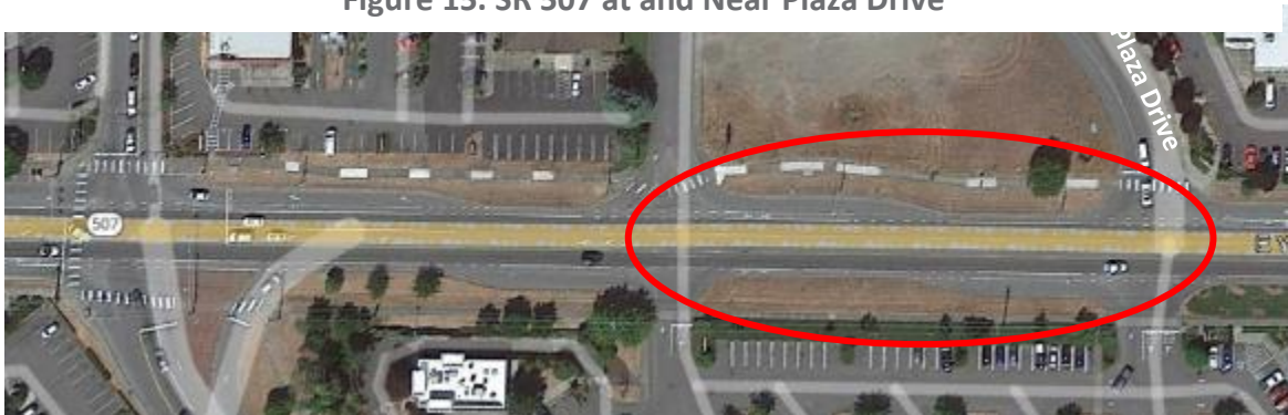
Figure 15. SR 507 at and Near Plaza Drive
