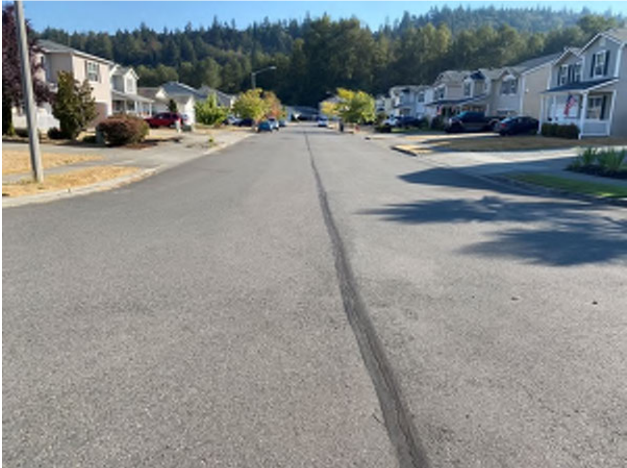
Figure 33. Crack Seal down Silvernail Street
