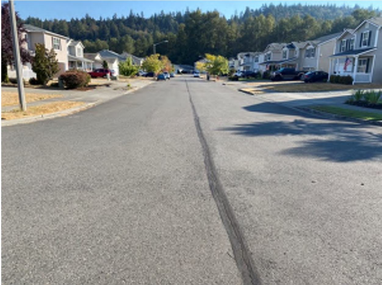
Figure 33. Crack Seal down Silvernail Street
