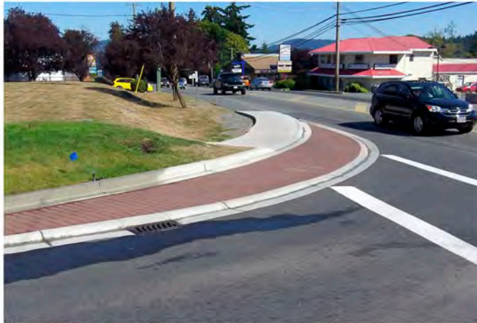
Mountable apron at Washington Avenue and Bridge Street
