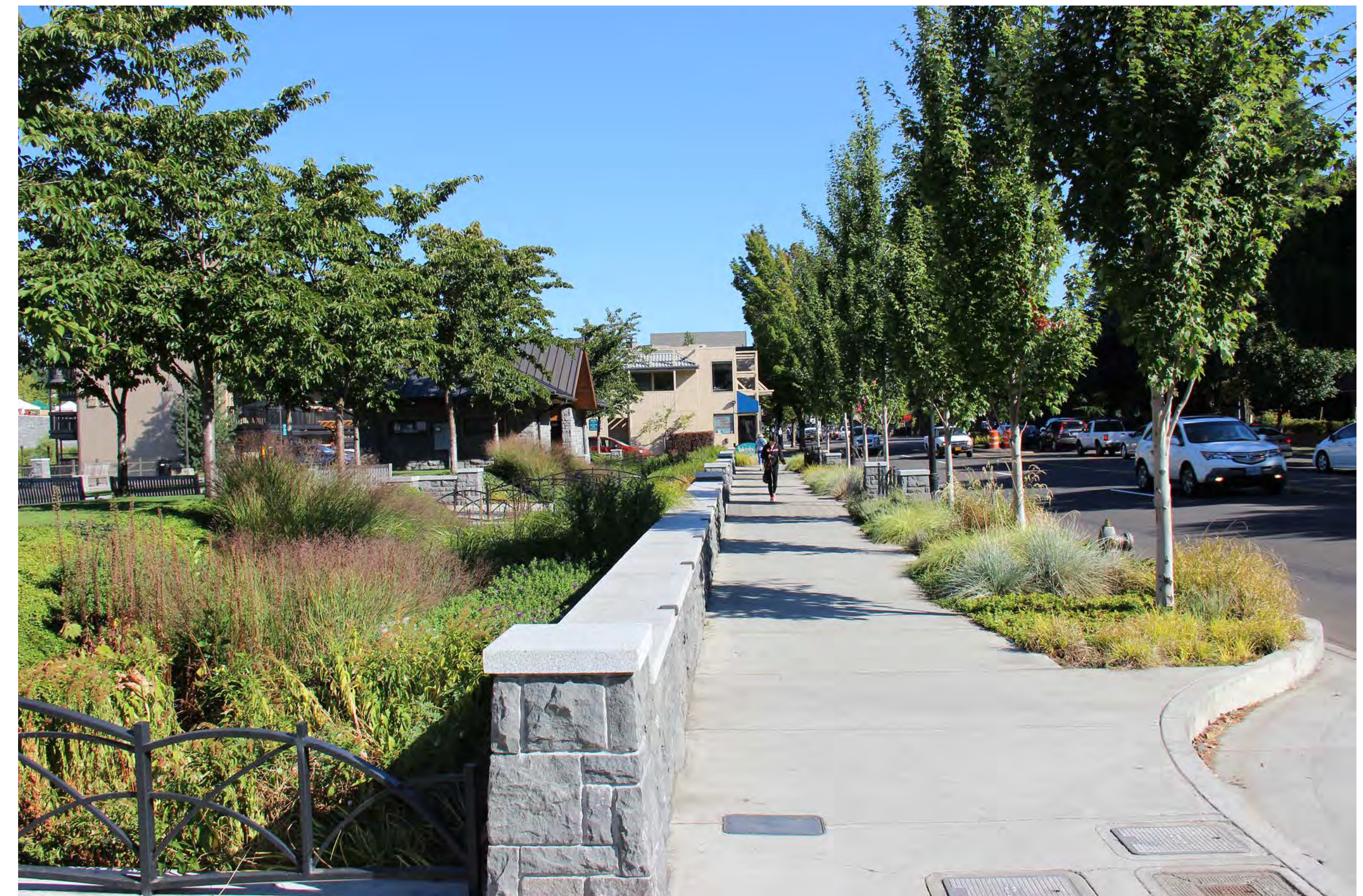
New sidewalk along Washington Avenue
