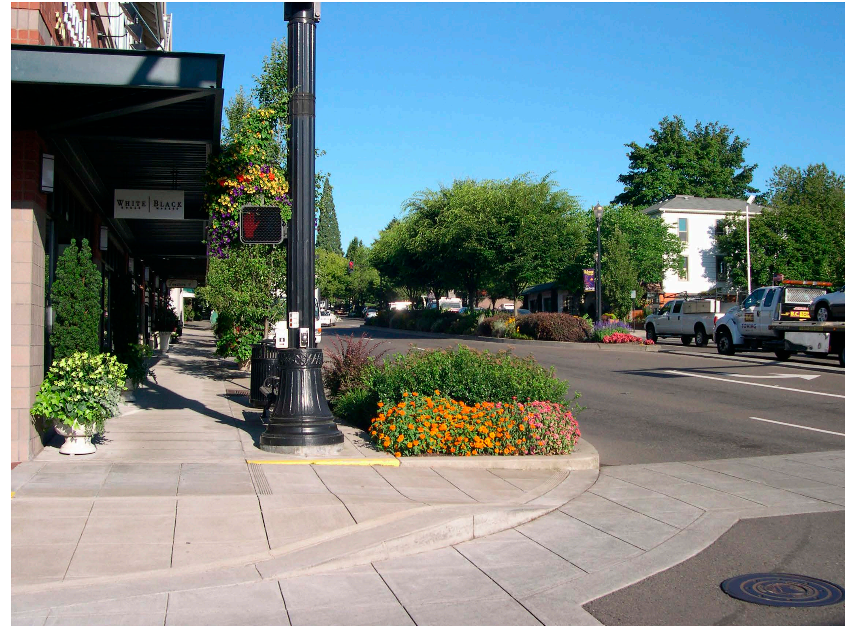
New curb extensions along Washington Avenue
