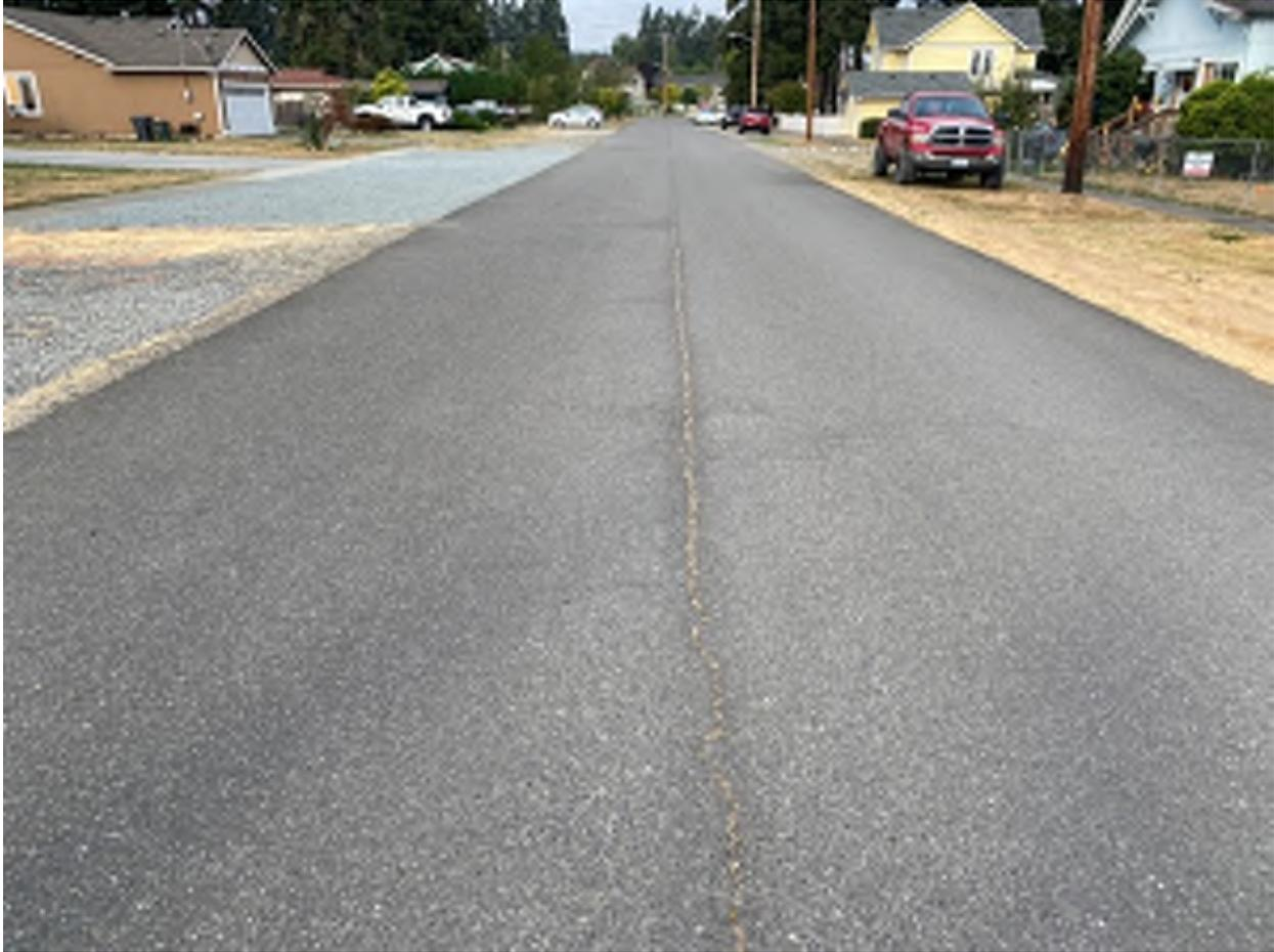
**Figure 15. Longitudinal Non-Wheelpath Cracking along Bridge Street**
