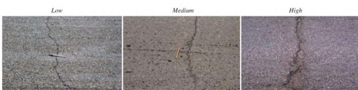
**Figure 17. Transverse Cracking Severities**
