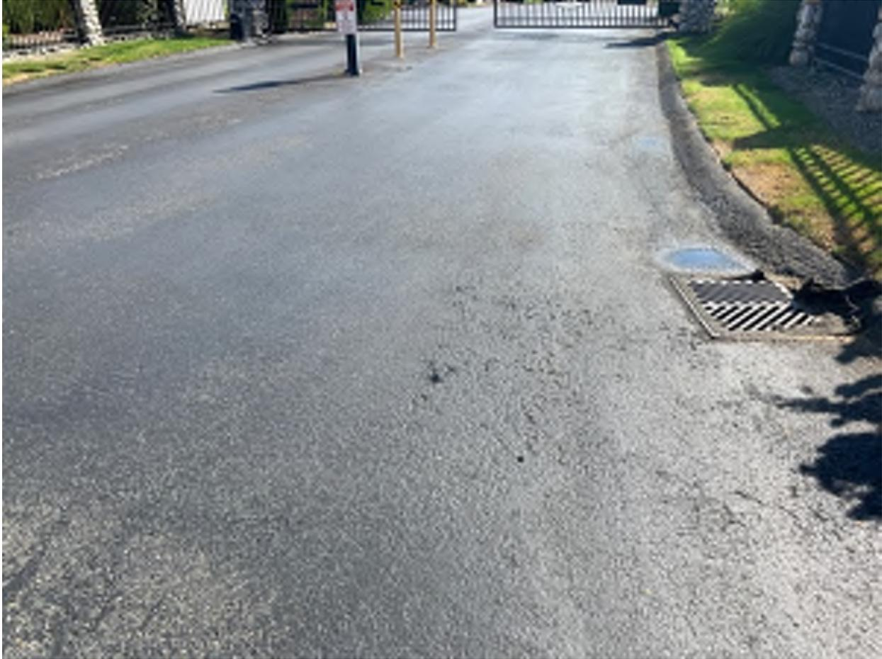
**Figure 24. Flushing and Bleeding on Park Place**
