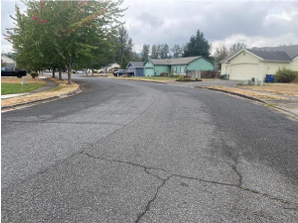
**Figure 18. Transverse Cracks on Belfair Avenue**
