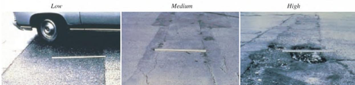
**Figure 26. Patching Severities**
