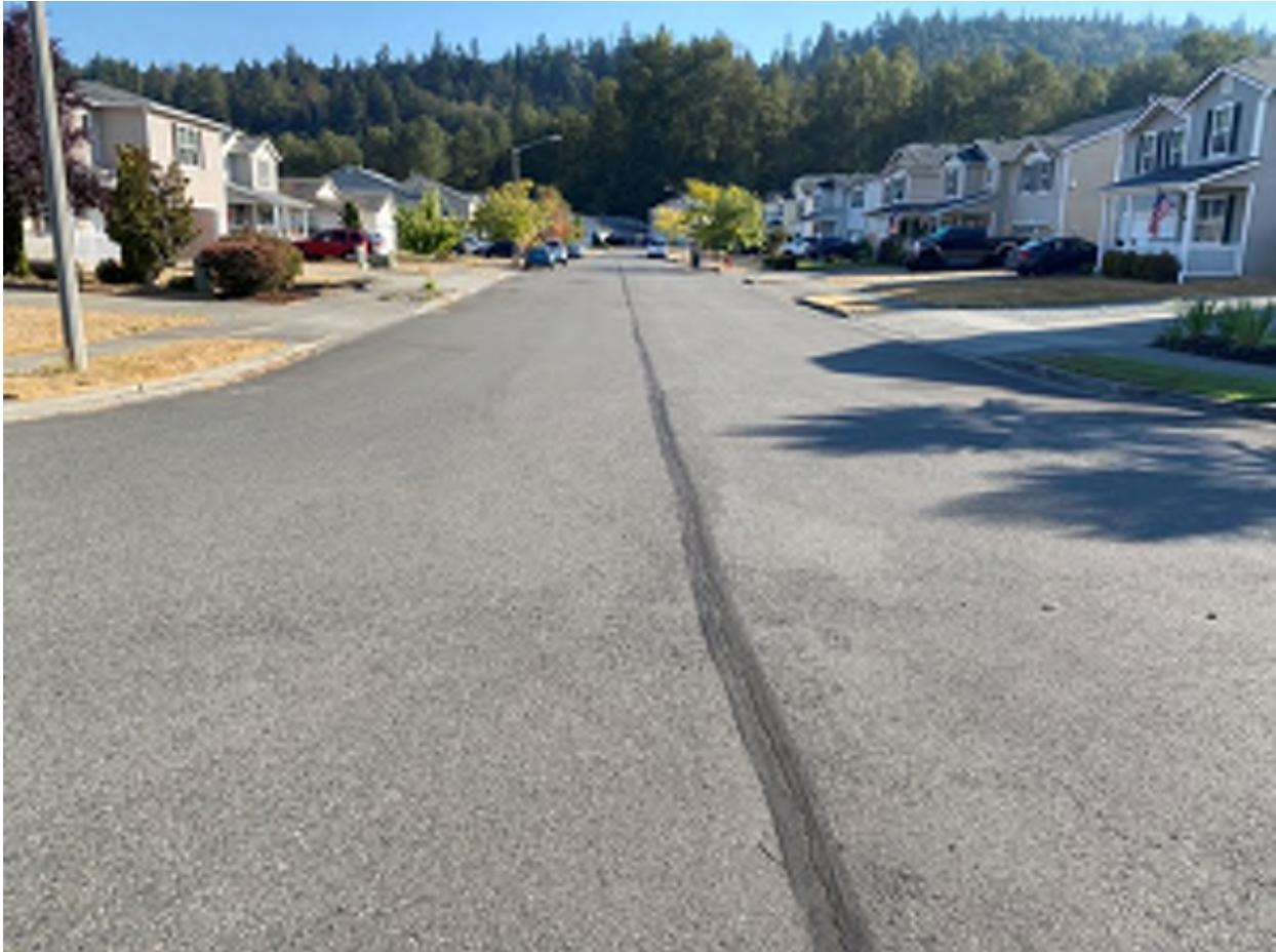
**Figure 33. Crack Seal down Silvernail Street**
