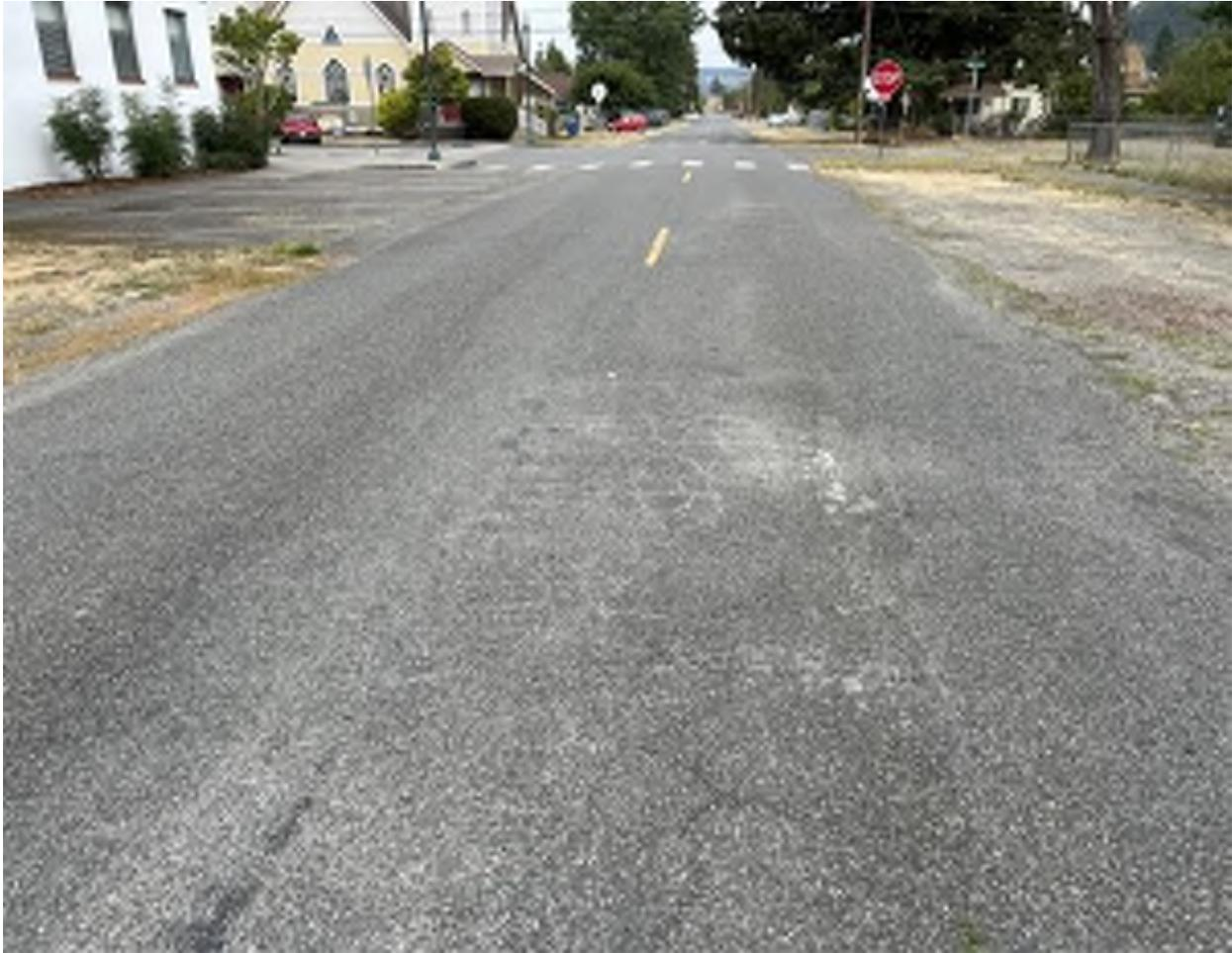
**Figure 9. Alligator Cracking on Varner Avenue**
