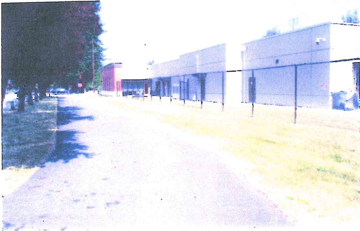
Picture # 5584 – Area of where the switch will be located.
