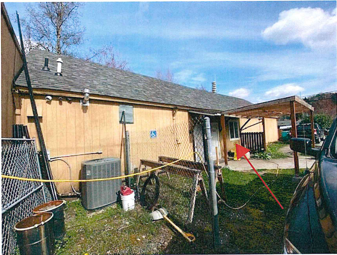
Existing condition, existing window seen under awning
