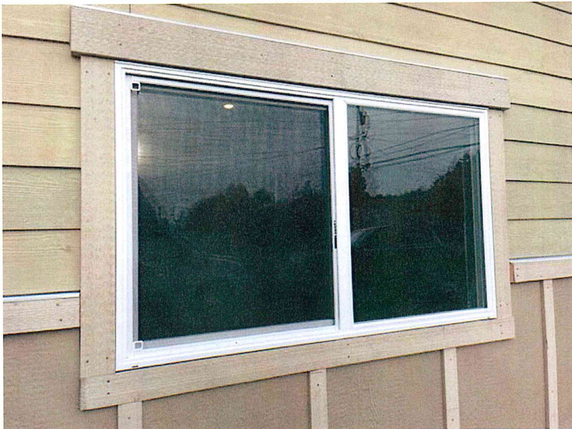
Proposed new window detail. Windows to match existing rear windows window trim detail to match previously approved front window detail
