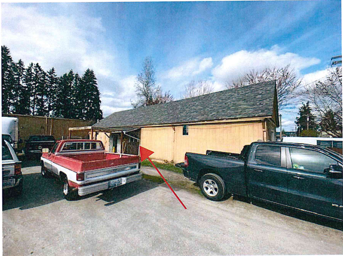
Existing condition, existing window seen under awning
