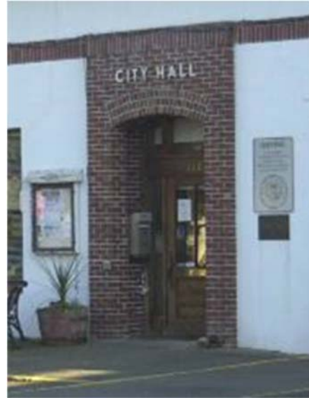
City Hall; 110 Train St SE.
