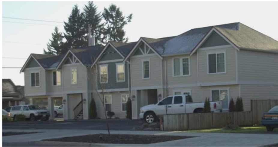
Five-plex Building; Corrin Ave SW and Bridge St SW.
