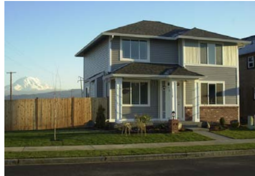
Village Green single family residence.
