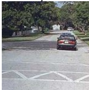
Ft. Lauderdale, FL – A 22-foot speed hump with zig-zag markings.
