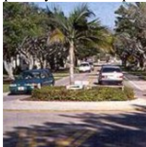
Ft. Lauderdale, FL – This traffic circle has a larger truck apron. Splitter islands and yield lines have been striped at each approach.
