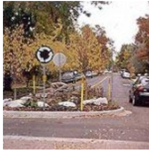
Boulder, CO – This traffic circle is combined with textured crosswalks. The center island uses low-maintenance landscaping.
