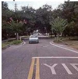
Sarasota, FL – This choker includes a yield line to alert approaching vehicles.
