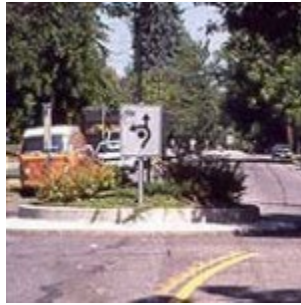
Seattle, WA – This traffic circle is located at a T-intersection. A truck apron is included that allows trucks to make a left-turn, while passenger vehicles are discouraged from using the truck apron by the short lip at its edge.
