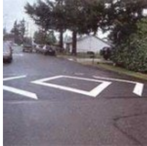
Portland, OR – This 14-foot speed hump uses a chevron marking pattern.
