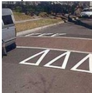
Charlotte, NC – This speed table uses stamped, colored concrete.
