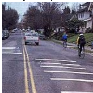
Portland, OR – This asphalt speed table uses leading horizontal stripe markings.
