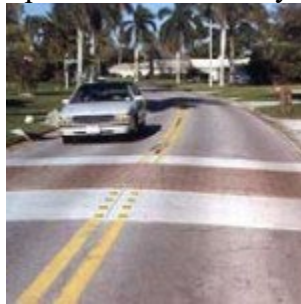
Naples, FL – This concrete speed table is combined with textured pavement to enhance its visibility and speed-reducing effect.
