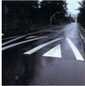
Bellevue, WA – This speed table is entirely asphalt with parabolic ramps.
