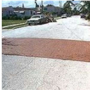
West Palm Beach, FL – This 12-foot hump is combined with Textured Pavement to enhance its visibility and speed-reducing effect.
