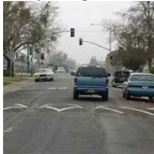
Sacramento, CA – This “speed lump” includes wheel cut-outs that allow buses and emergency vehicles to pass without slowing.
