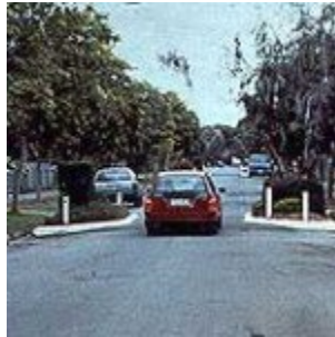
Howard County, MD – With one-lane chokers, vehicles on one side yield to vehicles from the other side until the queue is cleared, just as on one-lane bridges.
