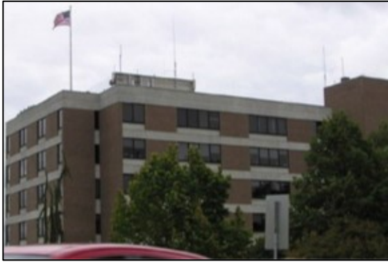
Acceptable Building-Mounted Macro Example
