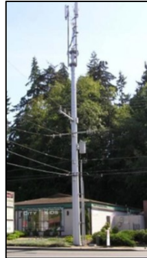
Unacceptable Structure-Mounted Macro Example
