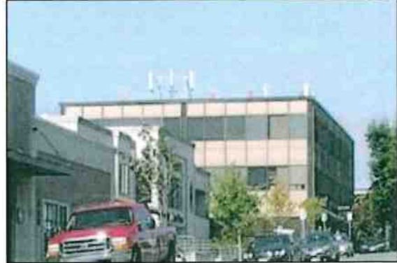
Unacceptable Building-Mounted Macro Example
