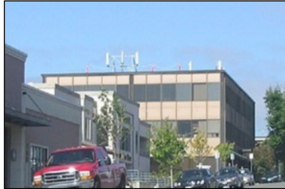
Unacceptable Building-Mounted Macro Example
