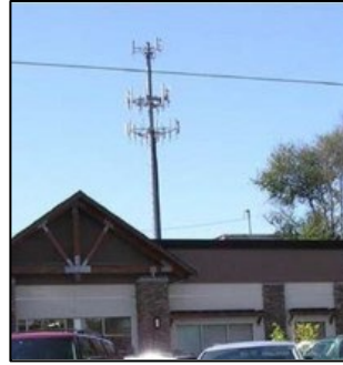
Unacceptable Monopole Macro Example
