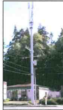
Unacceptable Structure-Mounted Macro Example
