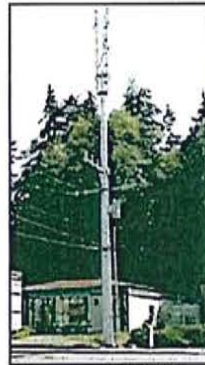
Unacceptable Structure-Mounted Macro Example
