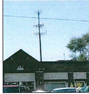
Unacceptable Monopole Macro Example
