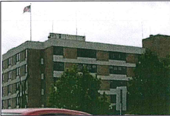
Acceptable Building-Mounted Macro Example
