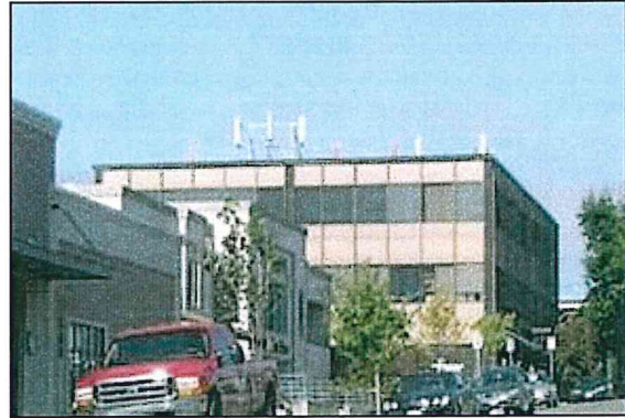
Unacceptable Building-Mounted Macro Example
