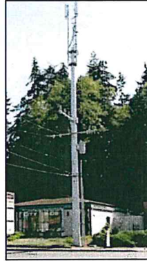
Unacceptable Structure-Mounted Macro Example
