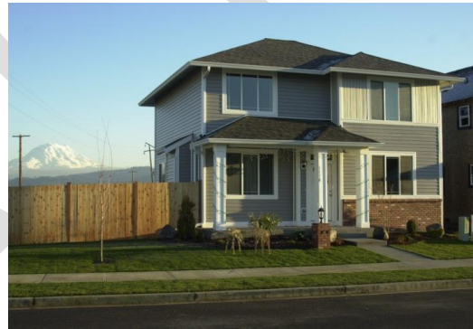
Village Green single family residence.
